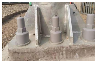
注油式螺栓防护套 Oil Filled Bolt Protective Cover
